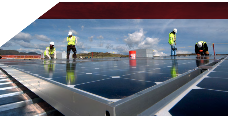
NREL. 2012. Solar Installation. Photo by Dennis Schroeder. 21512.
