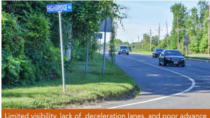
Limited visibility, lack of deceleration lanes, and poor advance signage at the intersection
